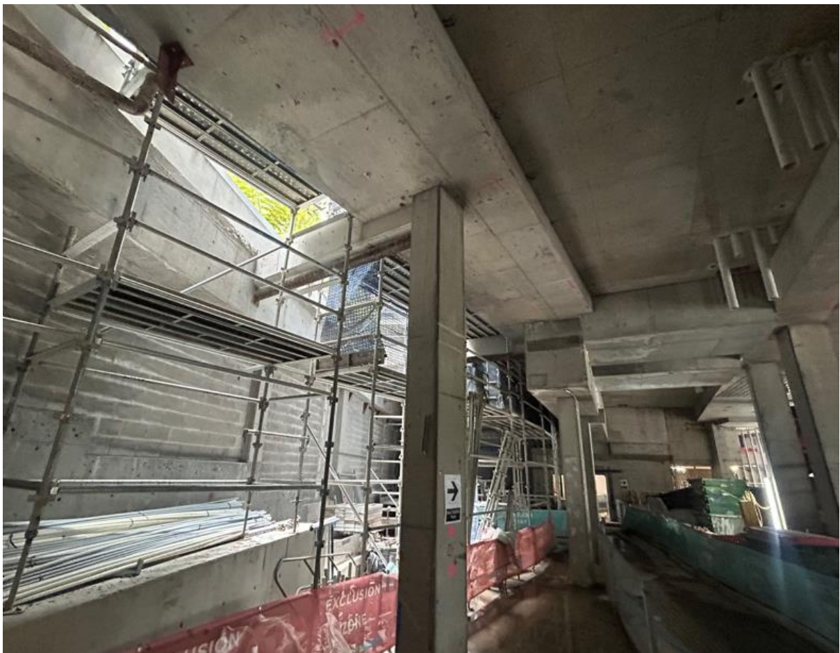
Figure 8: Existing 5-6 metre wall fronting a proposed terrace location (Lot 10) on the northeast side of the site, viewed from the ground floor facing northeast
